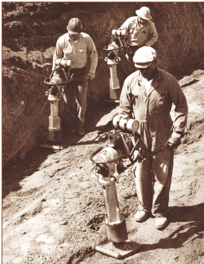
Wacker brothers' high speed GVR-100 rammer was a highly effective, one-man-operated machine that saved significant construction costs.
